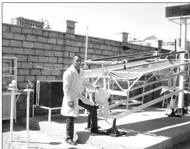
Figure 1. Solar plant with parabolic trough concentrator
